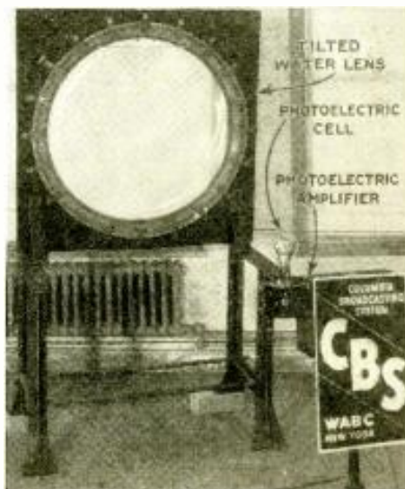
Fig. C Photograph of the receiving lens and the photoelectric cell used in the experiments.
